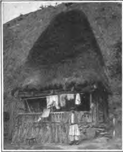
THE MOTZ PEOPLE—MOUNTAIN DWELLERS (The pointed, thatched roofs of their houses sometimes serve as snow-slides)
